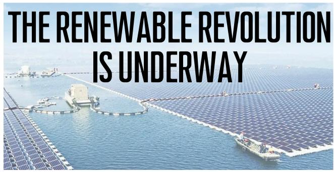
Floating on a lake over a collapsed coal mine, the power station in Anhui province in China can produce 40 megawatts of energy. (Smithsonian Magazine).
